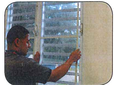
Install or repair window & door screens.
